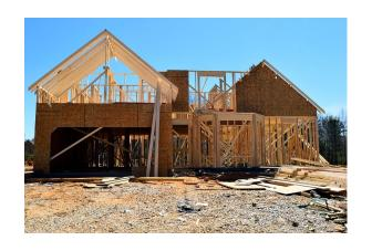
Members of the Department attended a course on how to identify wood frame construction and light weight building construction sites. Lightweight construction is generally considered to be either wood frame or steel building materials, where the roof and/or floor supporting systems are constructed of lightweight prefabricated materials. The members learn how to handle the hazards of these buildings during emergencies.
